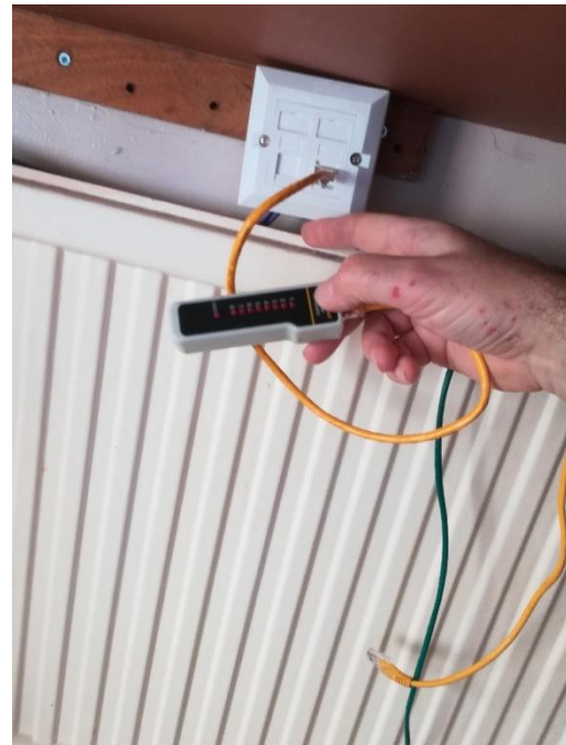
Test 2: Connectivity between patch port 2 to wall port 2
